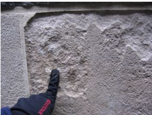
Eroded limestone
