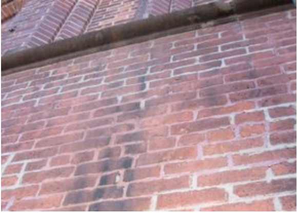
Atmospheric soiling on brick
