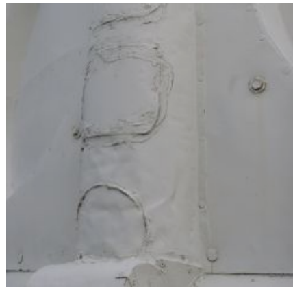
Sound patch repair in sheet metal
