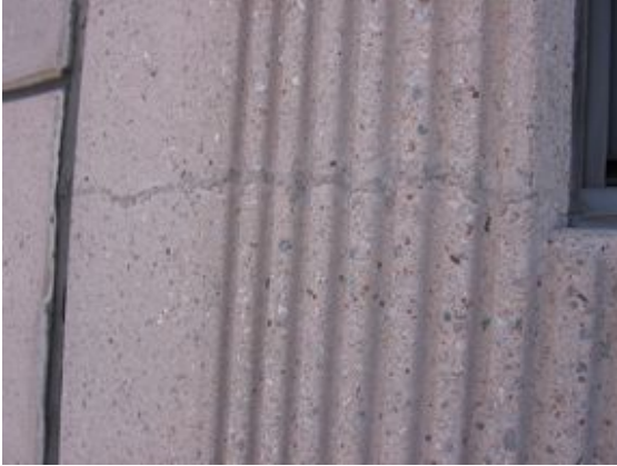
Sound crack repair in precast concrete
