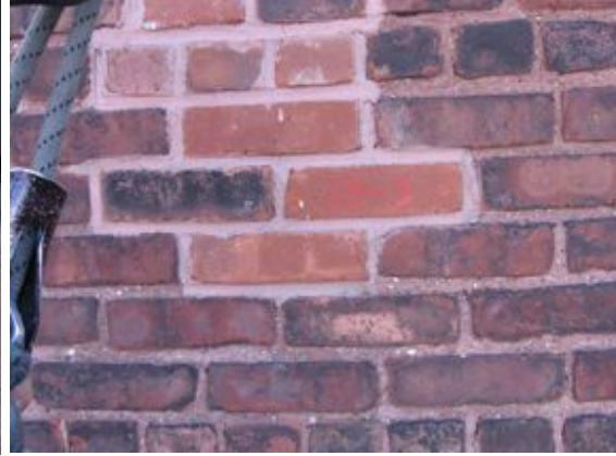
Replacement repair in brick
