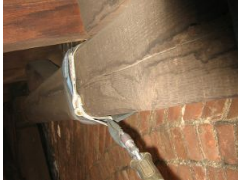
Checked structural wood member
