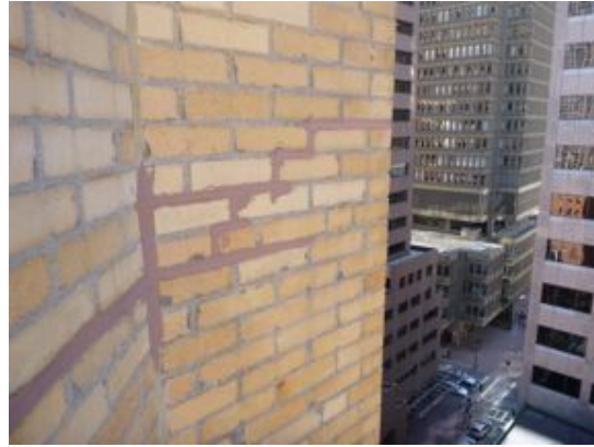
Caulked mortar joints in brick masonry
