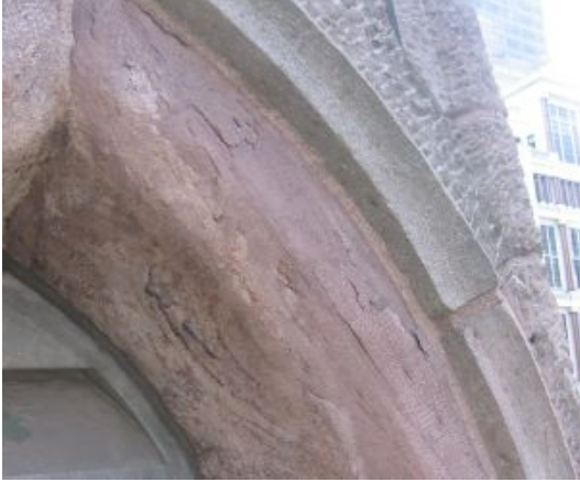
Delaminated sandstone
